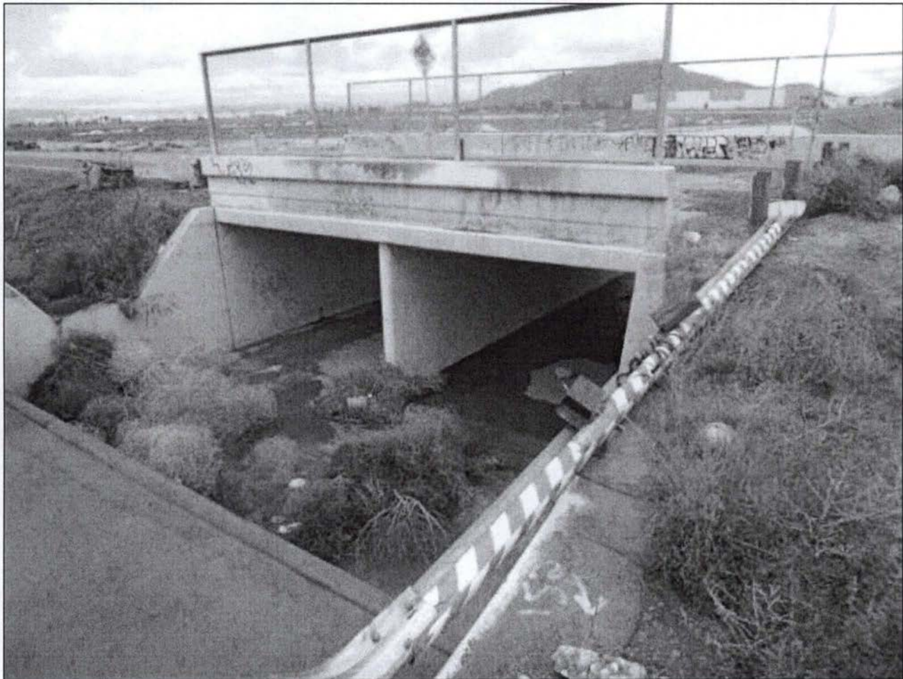
Figure 5. Double cell culvert on the west side of Webster Avenue (view to the northeast).
