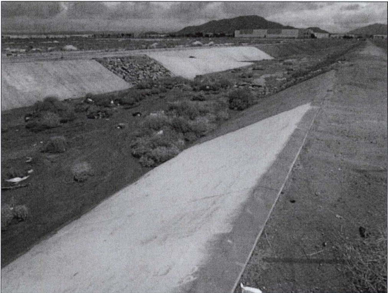
Figure 2. Lateral B-Oleander Channel immediately east of Webster Avenue (view to the east). Extensive improvements were made in 2004, including widening the channel, reconstructing and paving the sloped sides with concrete, and adding a strip of rip-rap paving.
