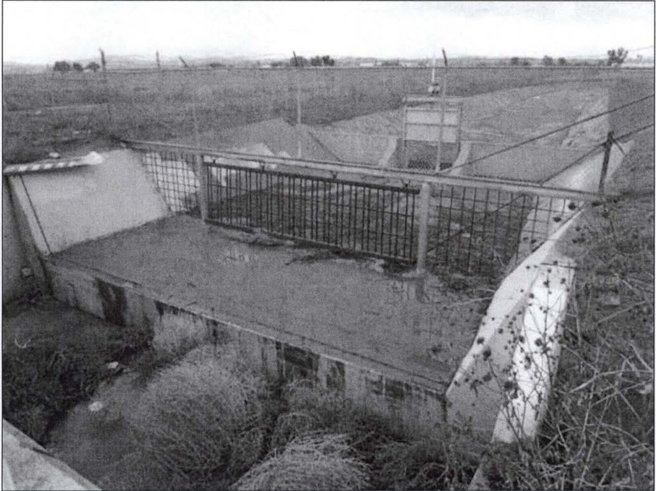
Figure 4. A concrete gate valve structure was constructed immediately to the west of the Webster Avenue culvert in the 1990s (view to the west).
