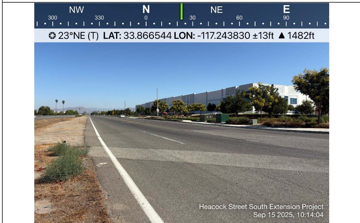
Photo 12: Site overview. View of northern portion of Heacock Street right-of-way, facing northeast.
