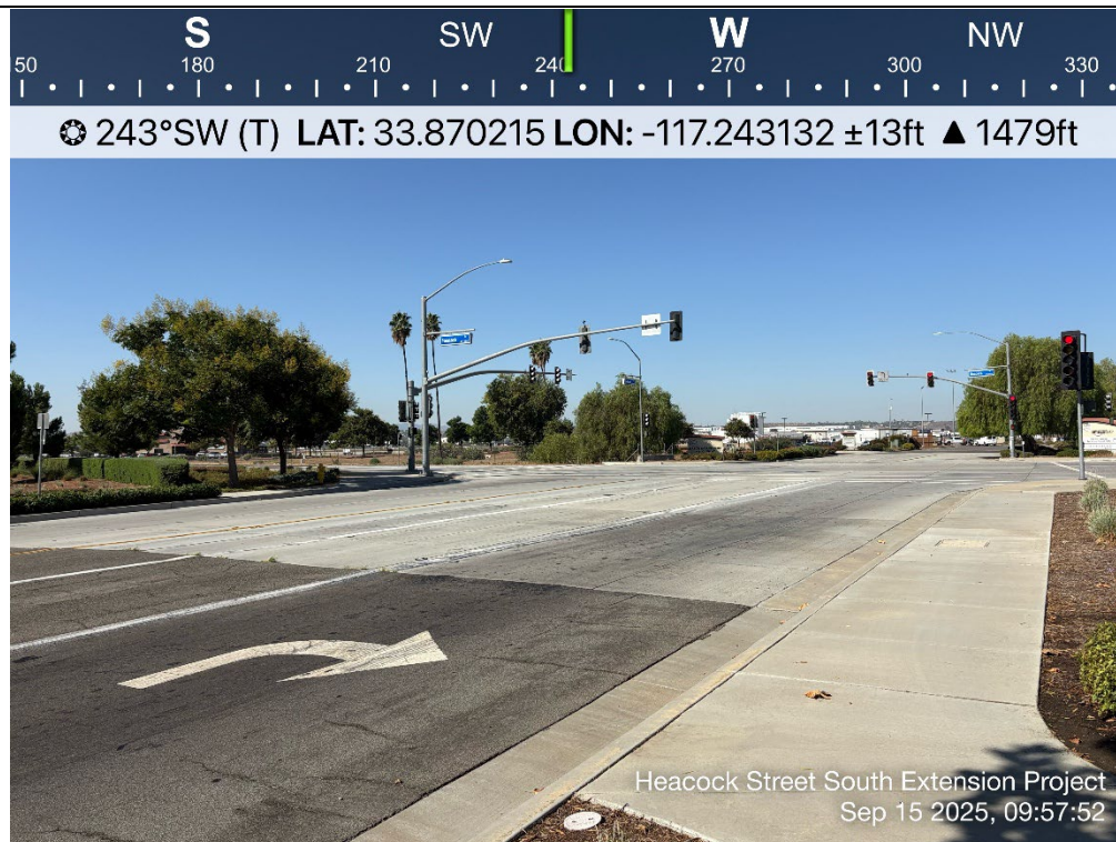
Photo 16: View of intersection of Heacock St and San Michele Road located near the northernmost part of the BSA, facing southwest.
