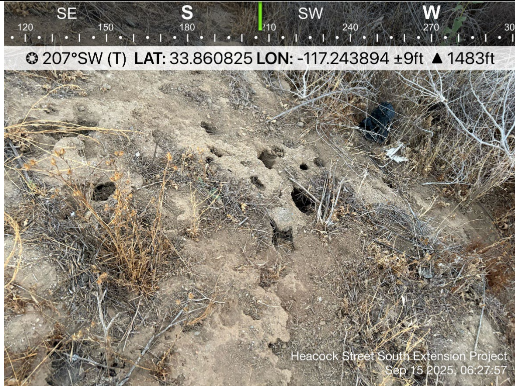
Photo 15: Small burrows seen throughout site. Majority of smaller burrows encountered within BSA were in deteriorated condition.
