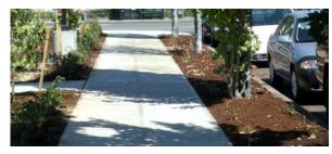
Low Impact Development practices like bioretention and porous paveing help retain groundwater and capture storm water runoff.
